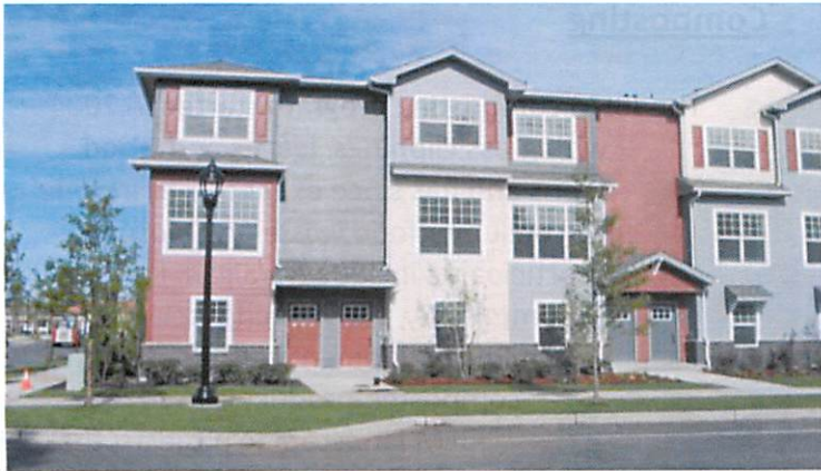
New duplexes in JBLM's Town Center provide a comfortable, urban living experience.
